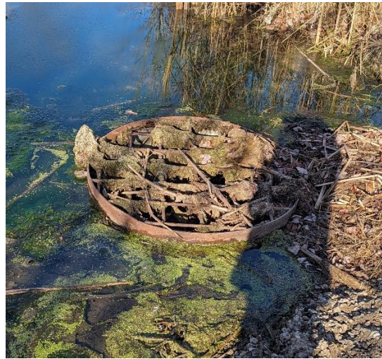
Figure 1: Drain in retention basin behind Creek Bend
